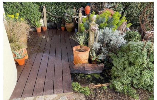
Brand new composite decking. Image: Geoff Stonebanks
