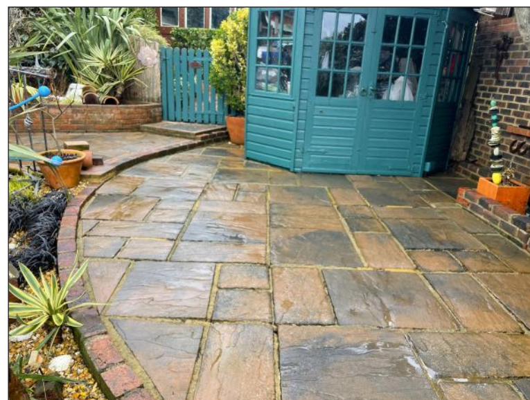
Newly power-cleaned paving
