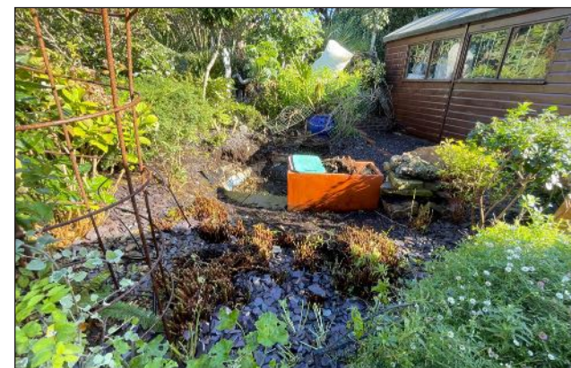
Ferns chopped back ready for steel wall
