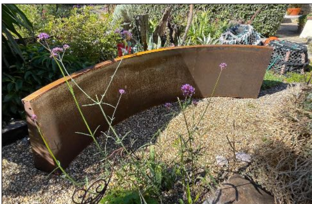
New corten steel wall delivered
