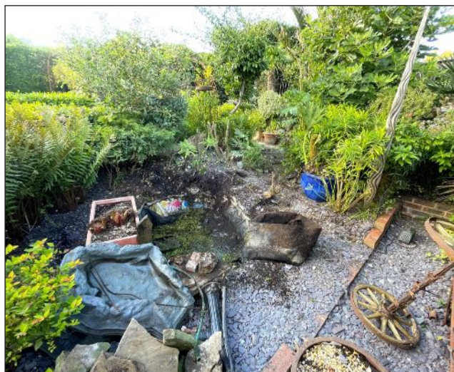
The area stripped ready for landscaping
