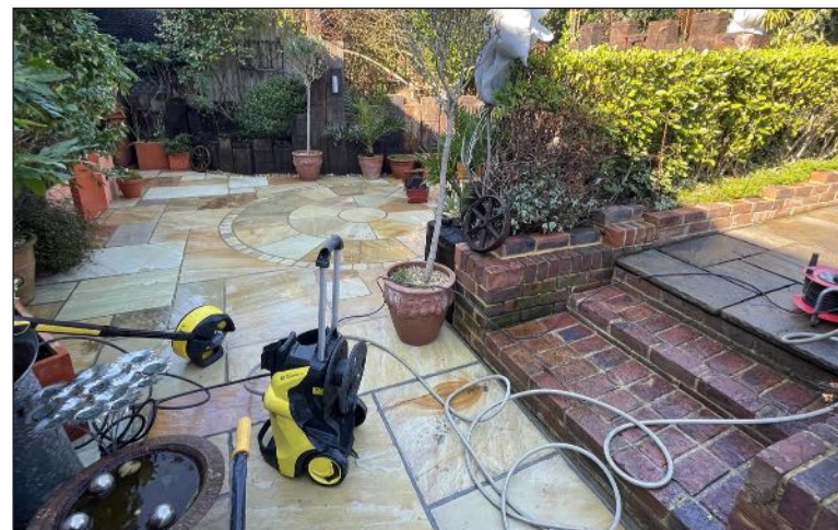
Pressure cleaning is now complete
